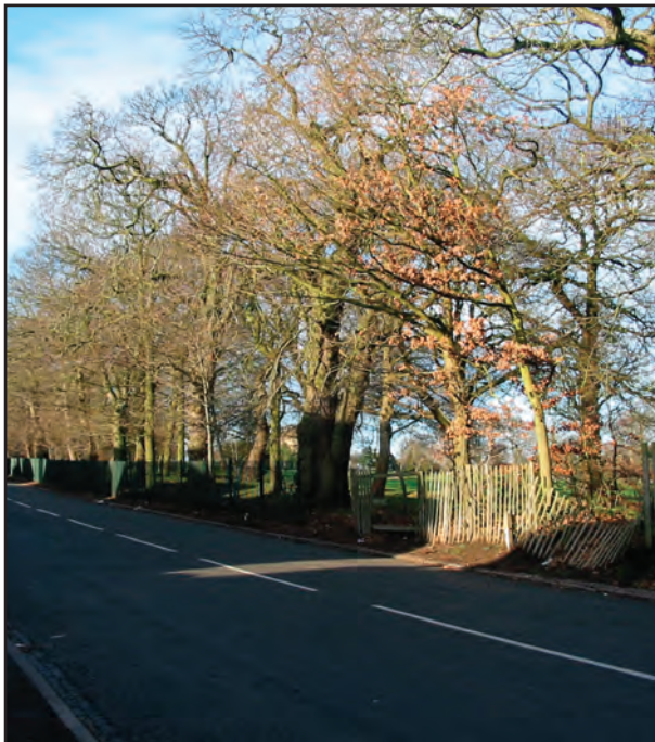
Railings being installed
